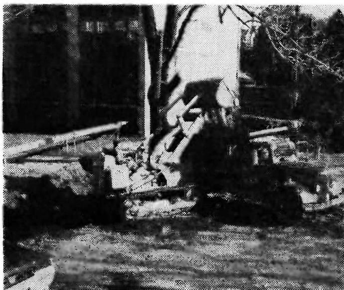
Moving excavator and pile bills with a diesel-powered tractor.
